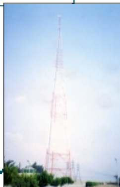
El Shabah 143 meter EEA Microwave Tower
