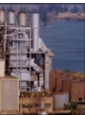
Cairo West 4x87 MW Steam
