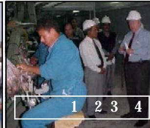
*Half tap splicing of feeder cable to transfer customers from existing Main Distributor Frame (MDF) to new MDF at Heliopolis Exchange vault room.*
